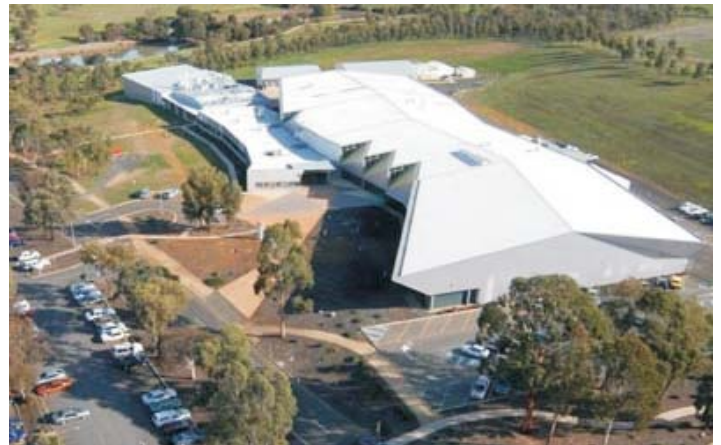
View of the current Geelong Technology Precinct building which houses Deakin University's light metals research and the ARC Centre of Excellence
